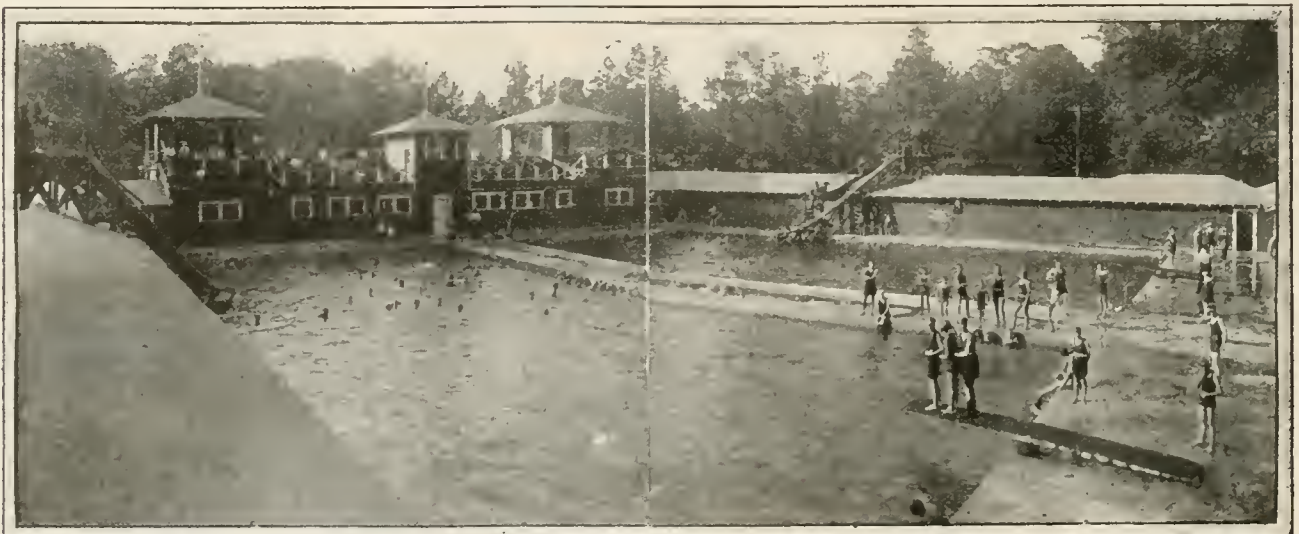
Two pools were built last summer and financed jointly by the city of Birmingham, Ala., and the Tennessee Iron and Coal Company. The pools measure 50x100 feet and have a capacity of 250,000 gallons each. The water is pumped through pressure filters and thence to ultra violet ray sterilizers, thus assuring a fresh, pure water supply at all times.
